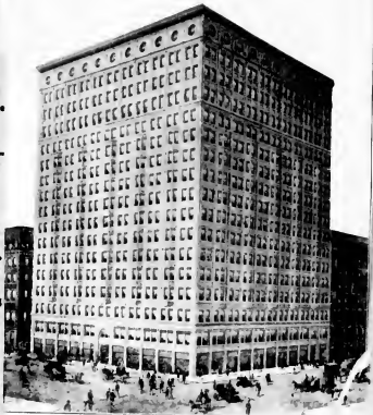
NEW RAILWAY EXCHANGE BUILDING, CHICAGO.
